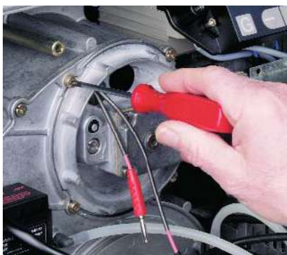
Loosening the mixing head
