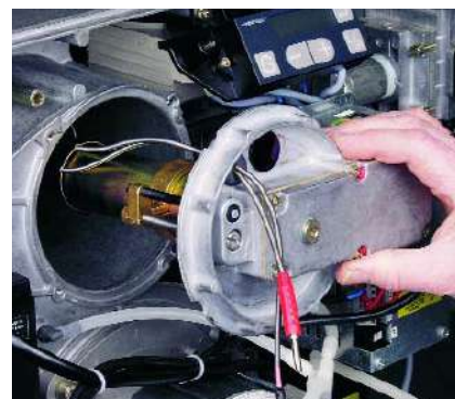
Removing the mixing head
