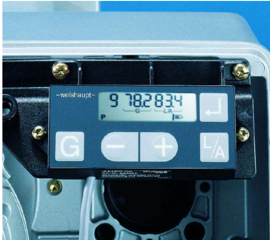
Burner display with all operating keys (burner cover removed)
